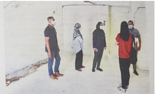
Homeowners taking a look at the cracks in a house in Jalan Taming Emas 3 in Sungai Chua, Kajang.
